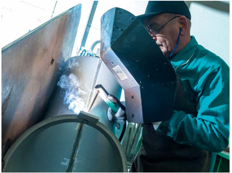
16” elbow in duplex 31803 welded at Petrol Raccord
